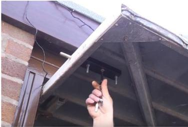
would be the case for garages having a connecting door to the house. The device is also only as strong as the ground into which it is bolted, and may not provide an effective enough deterrent on a paved driveway for example. In these situations it is best to install bolts to secure the door to the frame, on both sides. These are locked by means of a special key, which allows operation from either within or outside
